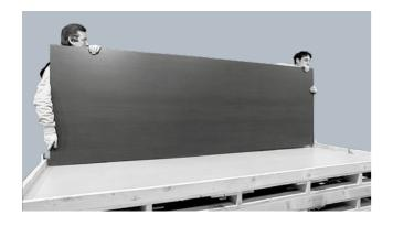
Guide the slab to its upright position, keeping it as straight as possible.
