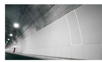
3plus, 5plus and 6plus Kerlite can be laid on curved surfaces, both concave and convex. Products with particular finishes can have certain limitations depending on the geometry of the slab, so please contact the Panariagroup Technical Department before proceeding with the installation.
