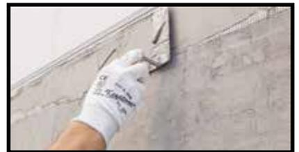
Position the profile and embed the mesh
