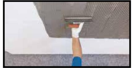
Spread the adhesive using a notched trowel vertically
