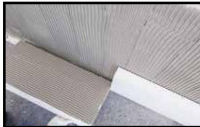
Installation of insulation panels with double buttering
